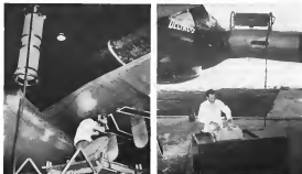
RADIOGRAPHIC SERVICE being performed (left) at Mitchell Air Base in a GE 179 is now suspended for welding leading edge of port by Raytheon X-ray and Metal Treating Laboratories Inc., of a wing. Radiographic position for inside wing. James W. King, New Canaan, L. I., in Connecticut, brought to equip machine; equipment (right) is typical set-up for X-raying wing spar.
